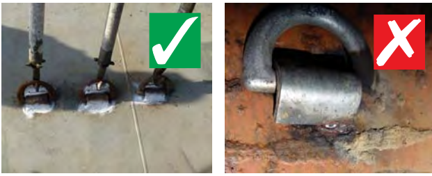
Examples of D-rings properly welded to deck (left) and poorly welded onto bulkhead (right).
