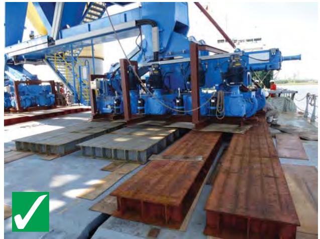
Load spreading 'mats' to protect the structure of the vessel.
